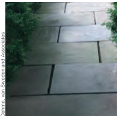
B 2 FEET X 3 FEET BLUESTONE BISECT PAVING
